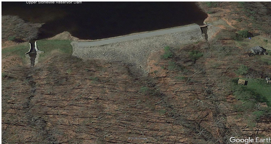
Fig. 15. Aerial view of the Upper Stoneville Dam (USA)
