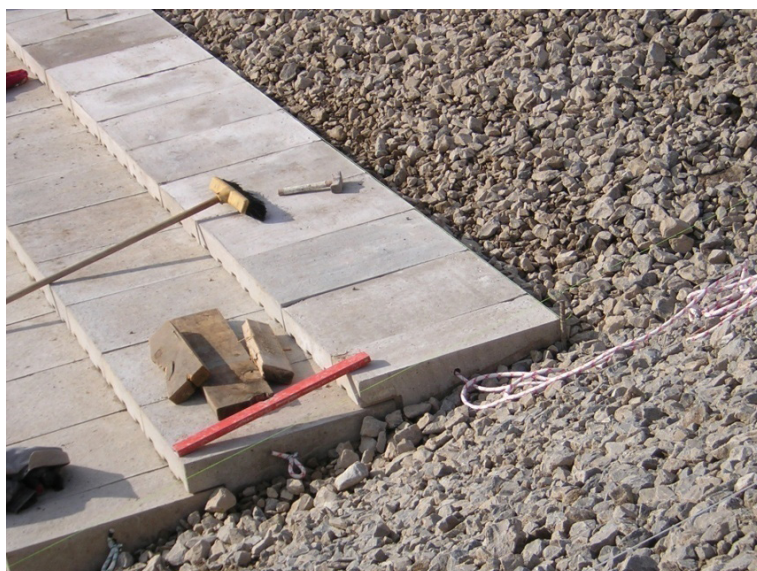
Fig. 30. Installation of wedge-shaped blocks in the spillway of the Barriga Dam
