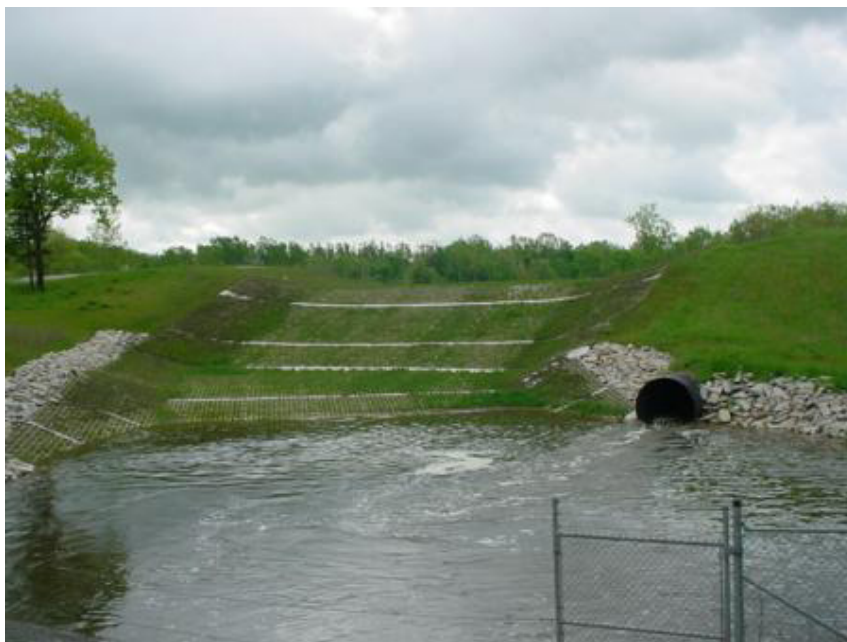
Fig. 8. Revegetation on articulated blocks (Photo: Clayton Fawcett, Contech Engineered Solutions)
