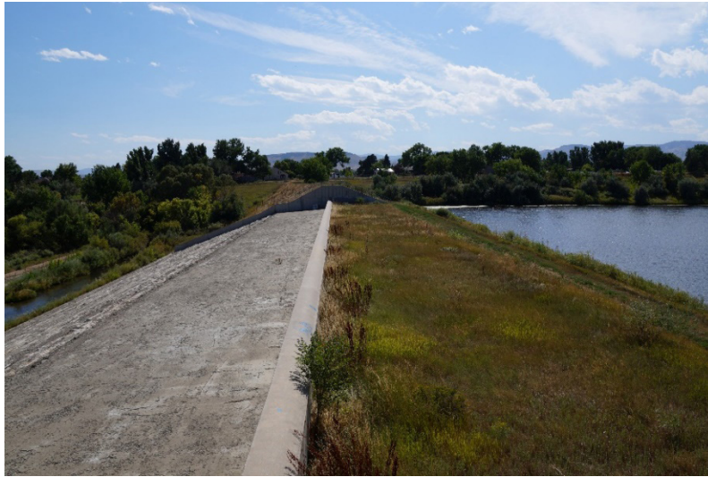
Fig. 3. Inlet area of the roller compacted concrete (HCR) protection of the Leyden Dam (USA). Protection on the left of the photograph and vegetation upstream face on the right
