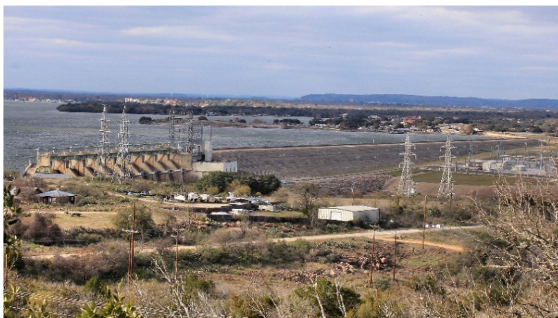
Fig. 33. View from downstream of the Alvin J. Wirtz dam with its slope protected with cement soil (Photo: Larry D. Moore, CC BY-SA 4.0, https://commons.wikimedia.org/w/index.php?curid=46264825 )
