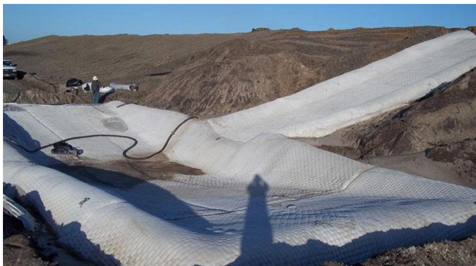
Fig. 11. Example of installing mortar-filled geocontainers in a chute ( https://synthetex.com/hydrotex/uniform-section/ )
