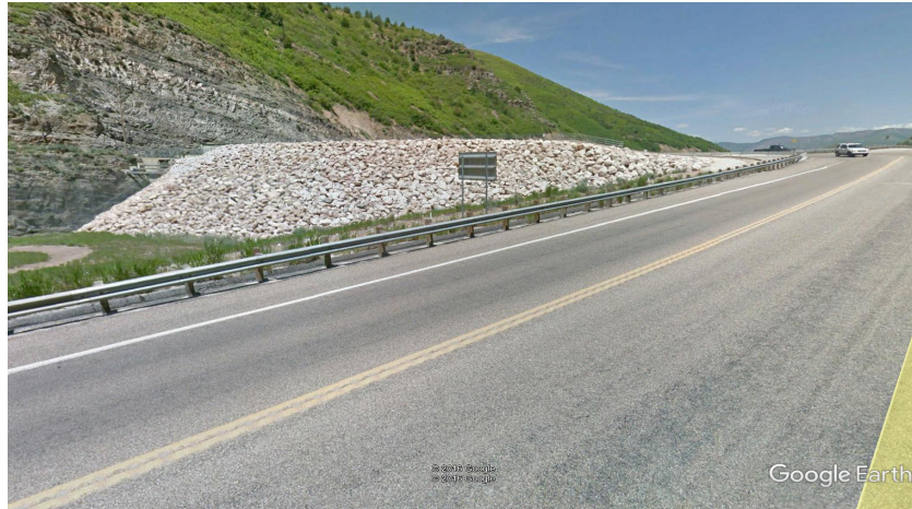
Fig. 17. View of the Pineview Dam (USA) (Google Maps)
