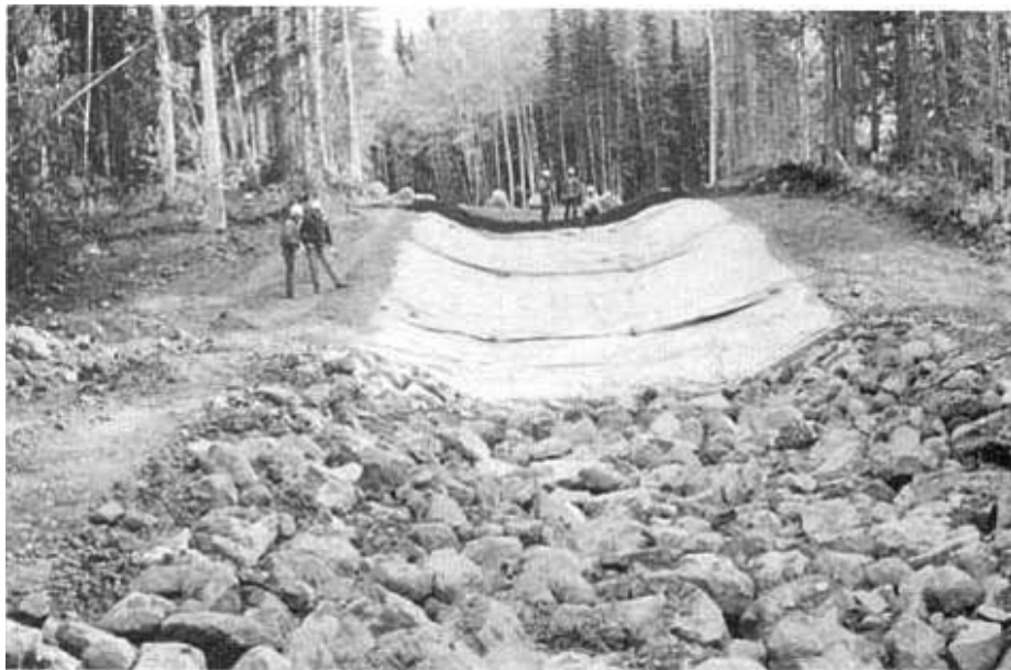
Fig. 9. Installation of the protective sheet at Cottonwood Dam No. 5 (Timblin, 1988).
