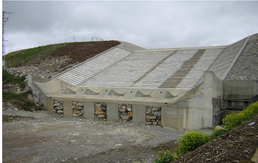
Fig. 5. Flip bucket for the wedge-shaped block spillway of the Barriga dam (Spain).
