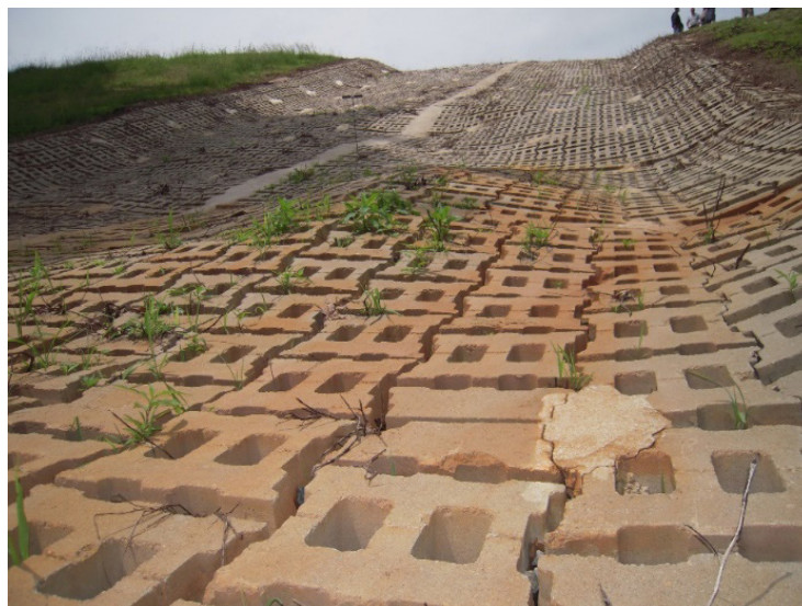
Fig. 31. Protection status with stitched CBAs of the No Name dam in the USA (Schweiger, Shaffer, & Nadeau, 2016)
