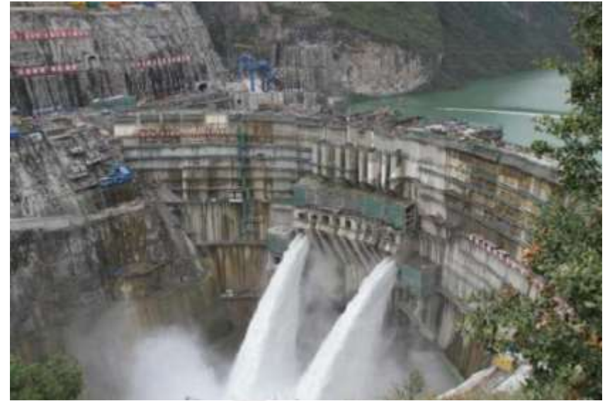
Jinping I (2013, H=306 m)
