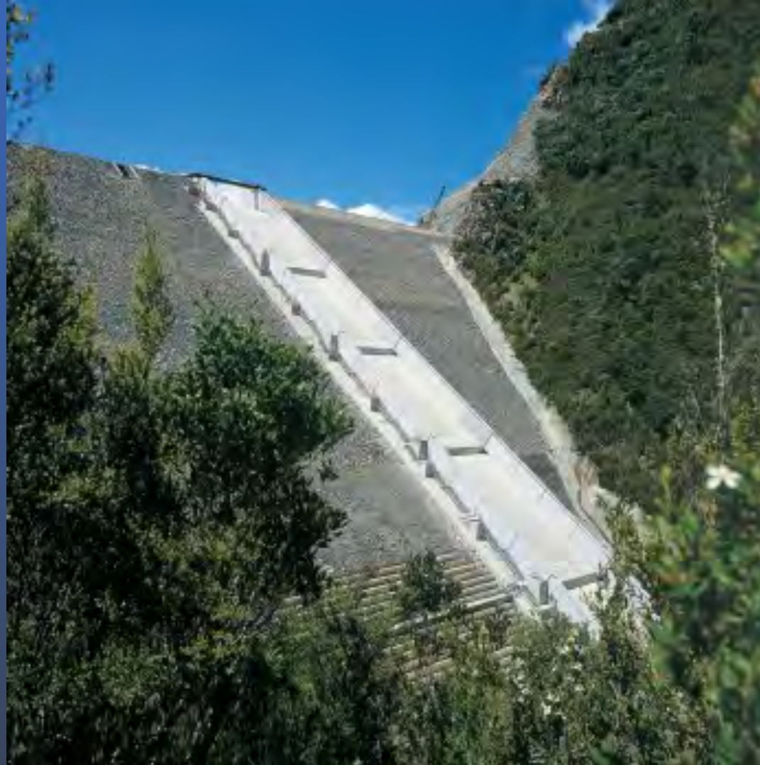
Presa de Crotty, Australia
